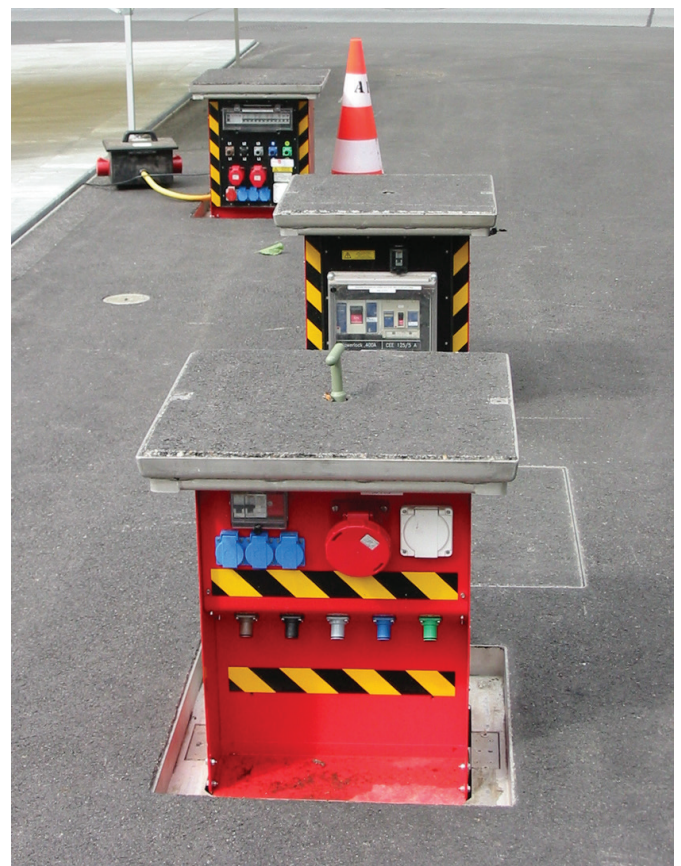
Telescopic, gas spring supported underfloor distributor system
